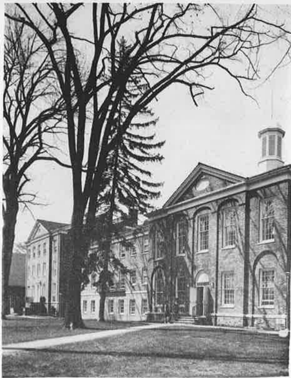
Coleman Hall is an example of Cazenovia College's fine architecture.
